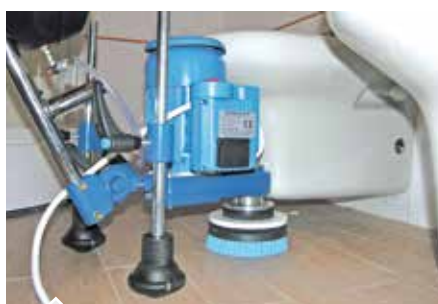
Works in tight spaces
