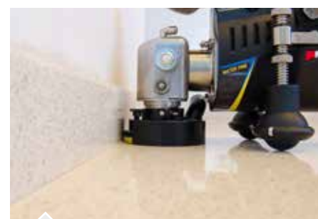
Grinding and polishing perimeters and edges.
